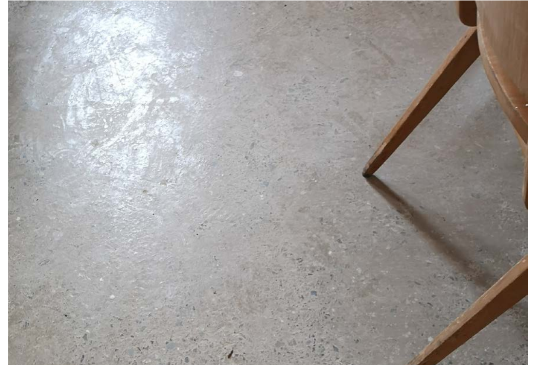
Figure 79. A polished and waxed rammed earth floor. Erden Werkhalle, Schlins.
