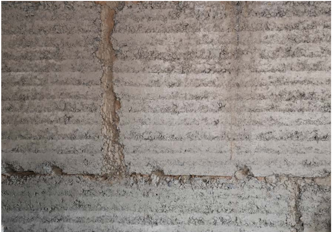
Figure 70. Stacked, but not yet retouched, rammed earth elements. Erden Haus, Schlins.
