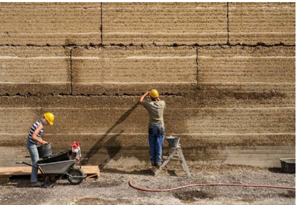
Figure 13. Retouching the joints to create a seamless monolithic appearance.
