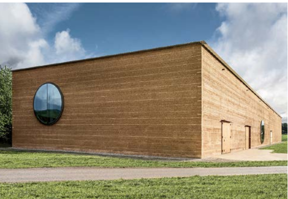
Figure 14. The finished result of the Ricola Herb Centre, made from prefabricated elements.
