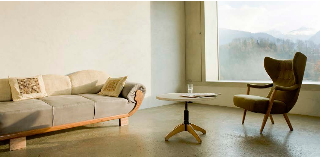
Figure 21. A finished rammed earth floor in Haus Rauch, similar to how a polished concrete floor can look, but with more texture.
