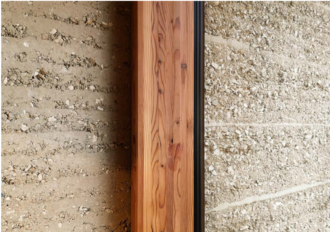
Figure 64. Interior and exterior. Swiss Ornithological Centre, Sempach.
