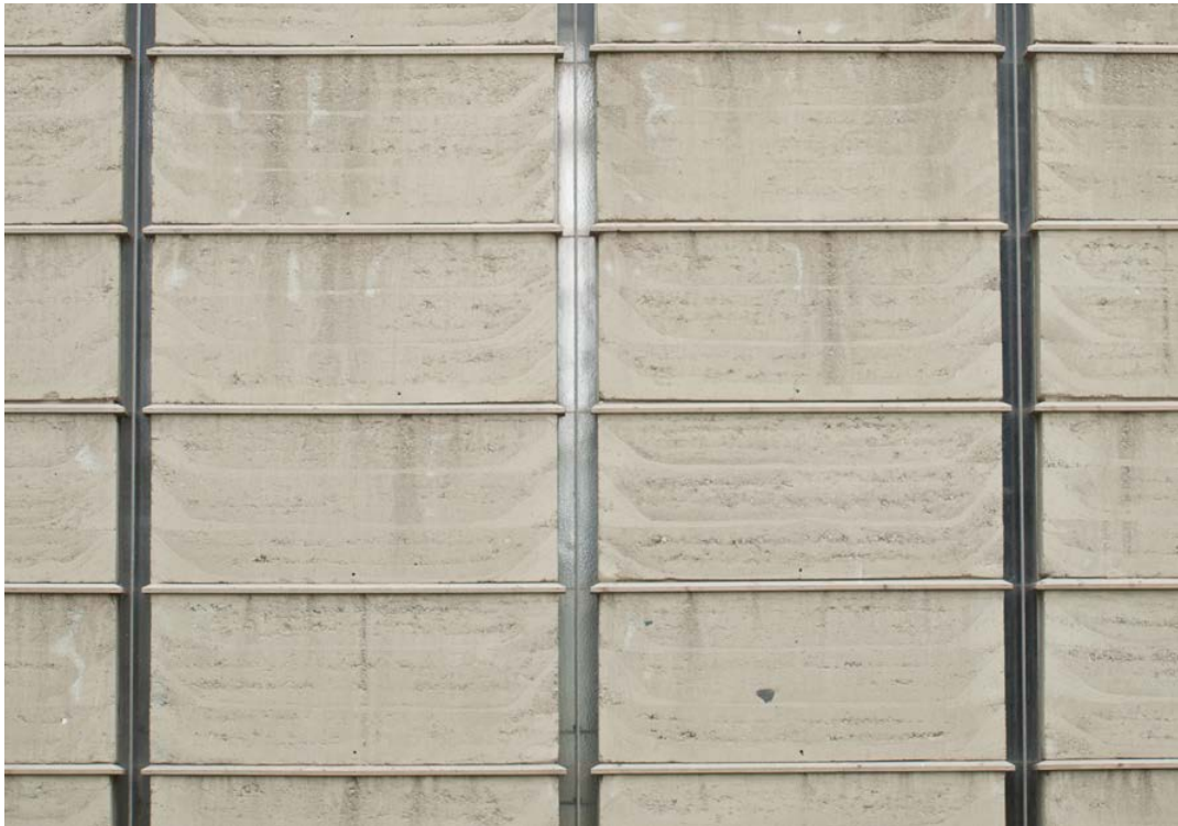
Figure 74. Instead of retouching the joints they have been emphasised with windows and wooden erosion checks here. Kiln Tower, Cham.
