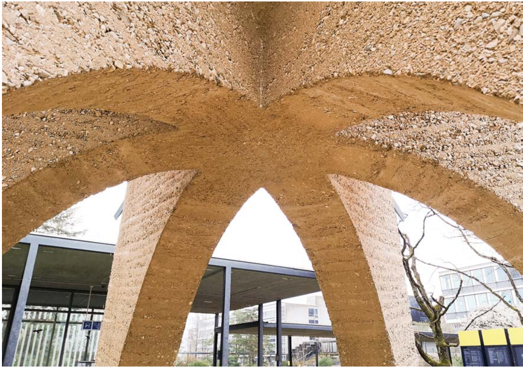
Figure 73. The rammed earth elements can be prefabricated in any shape and joined seamlessly. ETH Earth Dome, Zürich.
