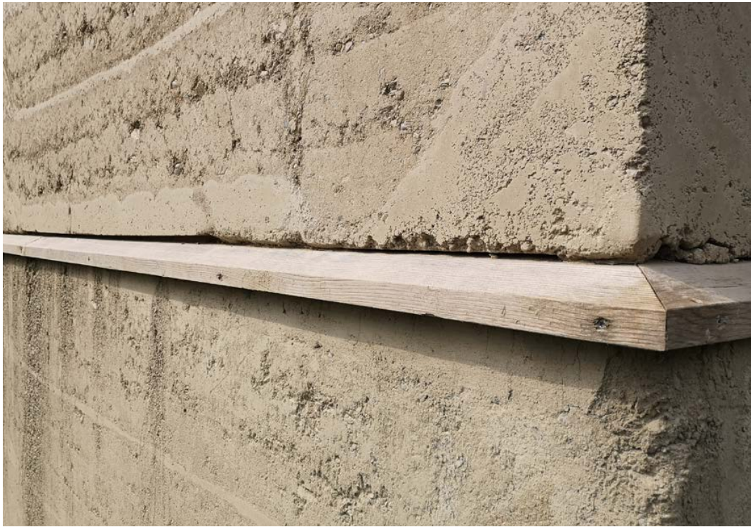
Figure 75. The wooden panels that these elements where prefabricated on were kept as erosion checks. Kiln Tower, Cham.
