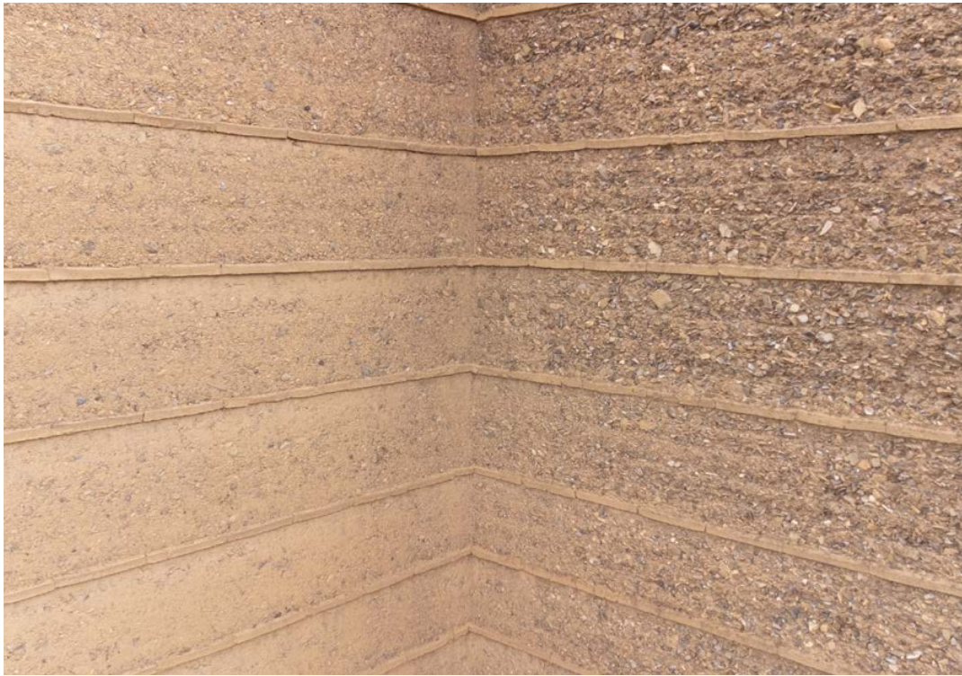
Figure 65. The general wind direction has caused more erosion on one side of the facade. Haus Rauch, Schlins.
