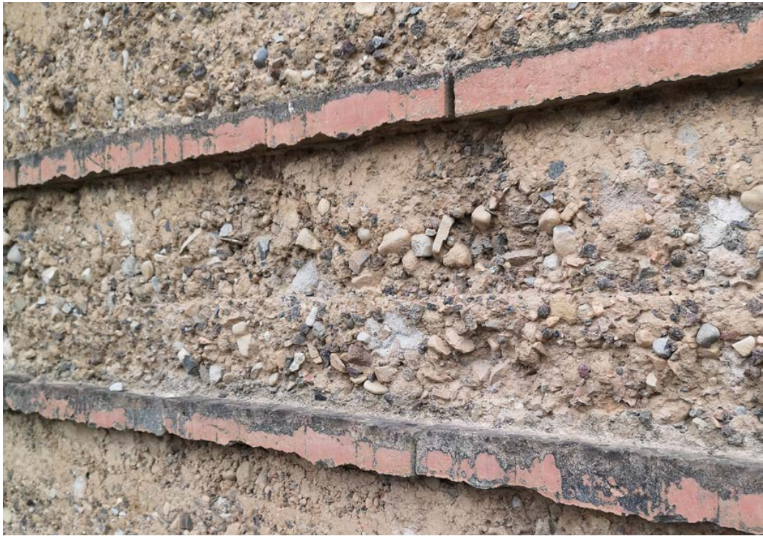
Figure 63. 30 year old exterior facade with erosion checks. Studio Rauch, Schlins.
