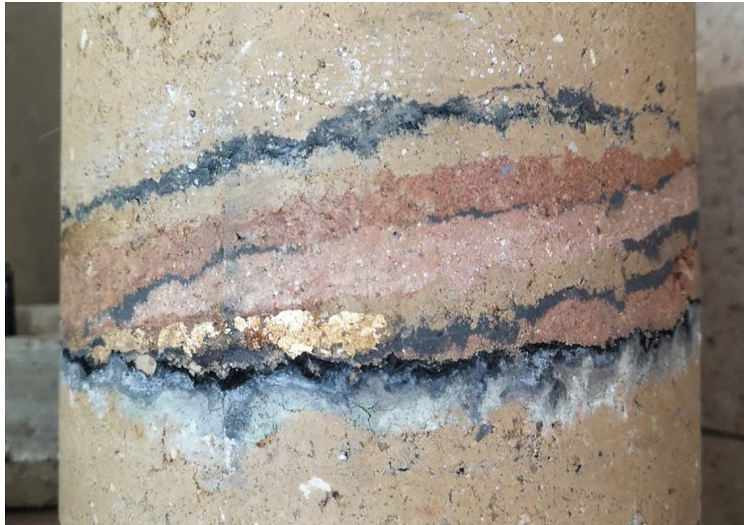
Figure 87. Different pigments and infills can be integrated in the rammed earth. Studio Rauch, Schlins.
