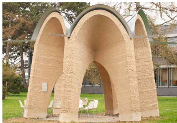
Figure 15. The ETH Cupola is a compression-only structure.
