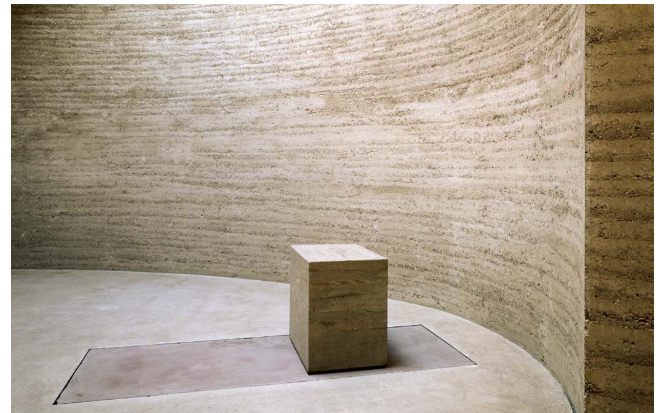
Figure 8. The Chapel of Reconciliation in Berlin, 1999-2000, is the first load-bearing rammed earth structure built in Germany for 100 years (Erden, 2000)
