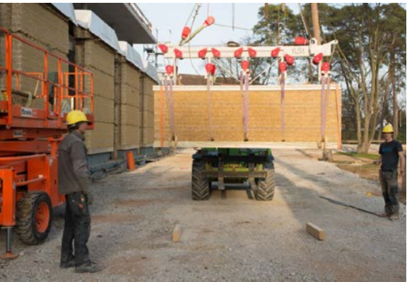
Figure 12. Lifting the elements on place with a crane.
