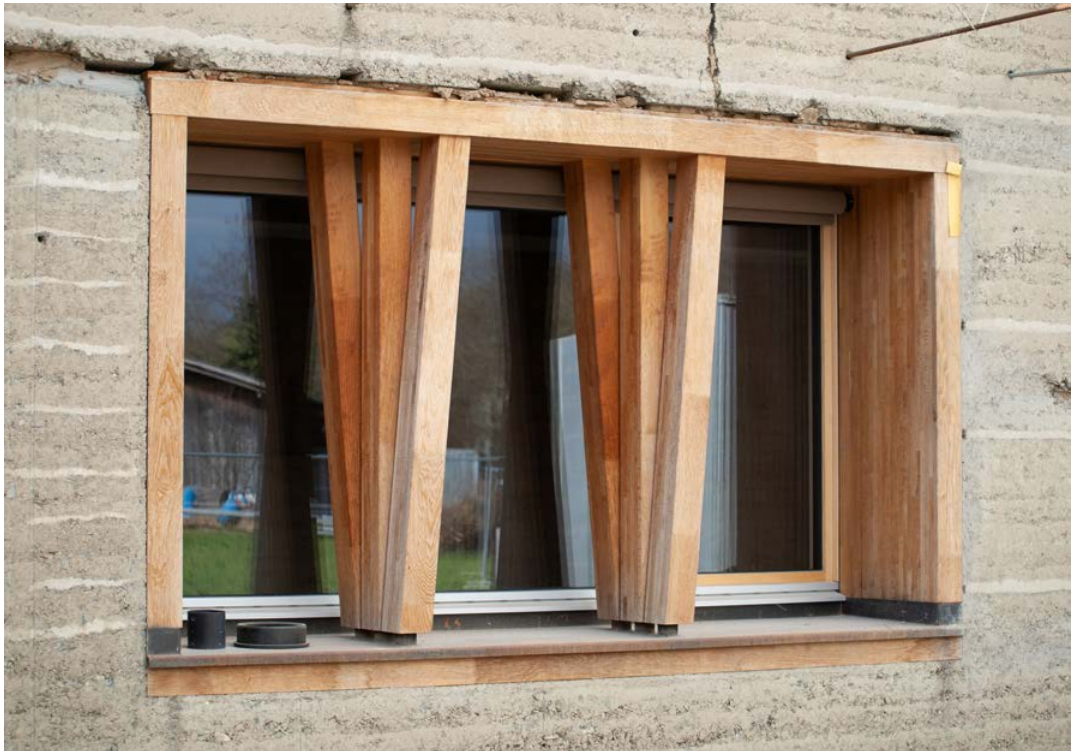
Figure 85. Instead of having a lintel beam above the window the whole frame is acting as a beam itself. Erden Werkhalle, Schlins.
