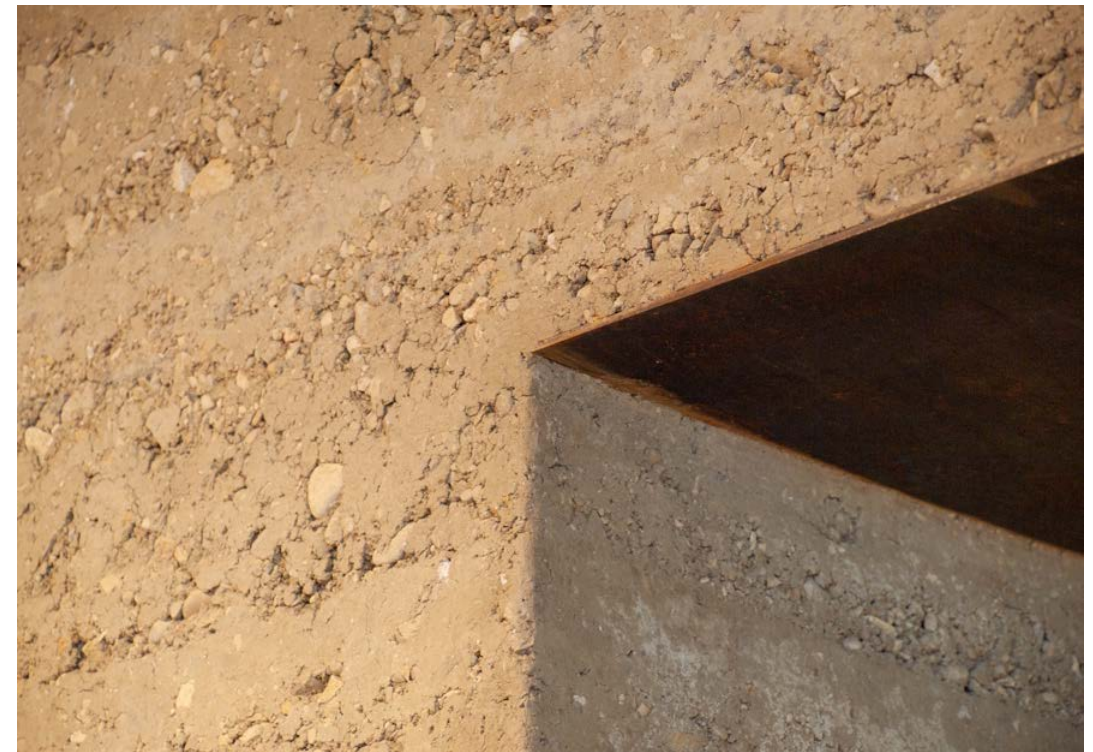
Figure 82. A thin metal plate seems to support the earth above, but a lintel beam is hidden behind. Swiss Ornithological Centre, Sempach.
