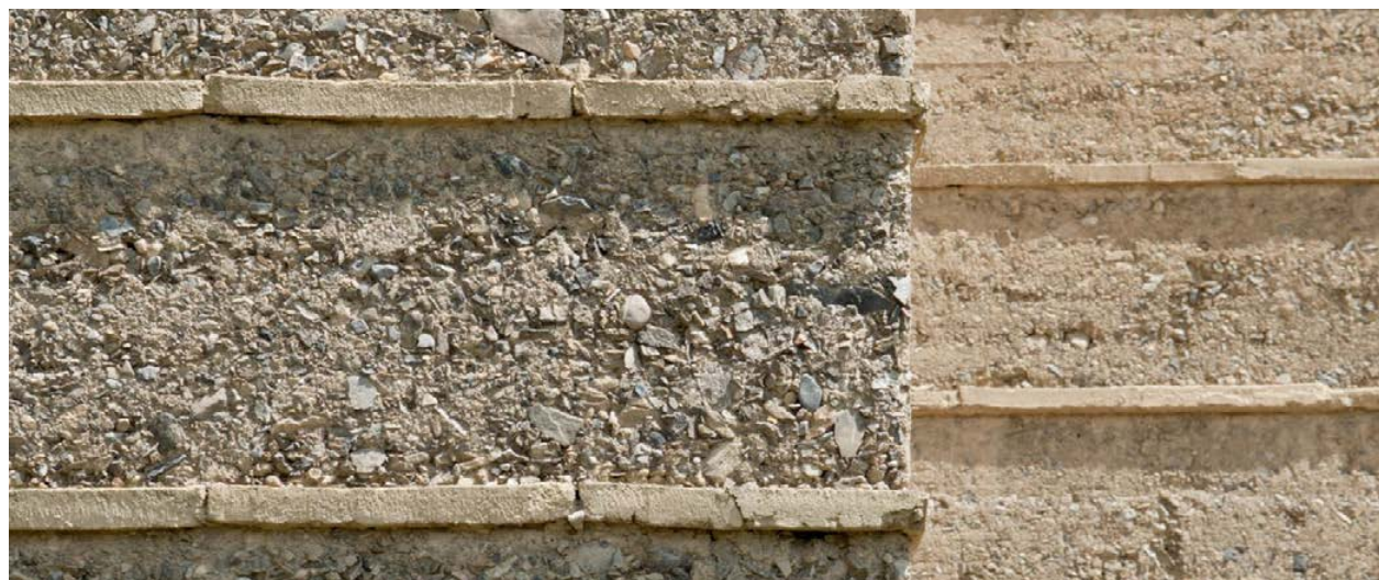
Figure 19. The smaller particles will wash away and reveal the stones, like this facade on Haus Rauch.
