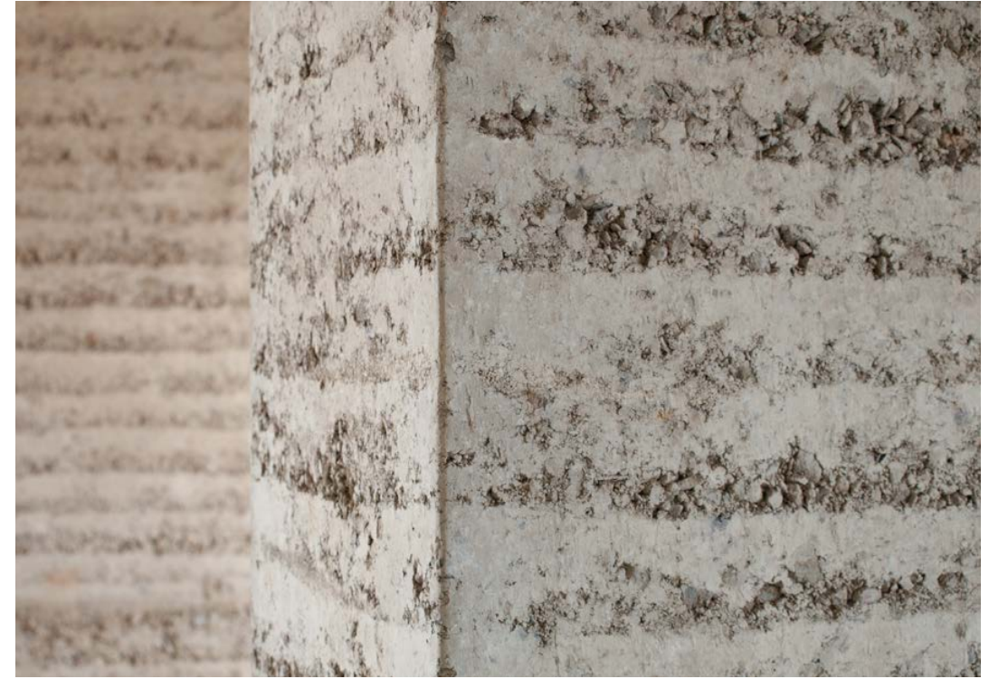
Figure 81. A retouched corner on an interior rammed earth wall. Erden Haus, Schlins.
